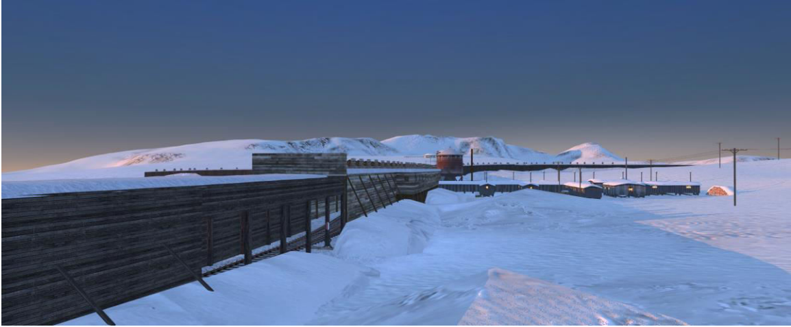
Corona Huge Snow Shed Complex Depot, Workshops and Housing
