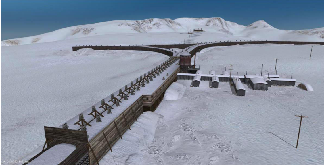
Corona Snow Sheds and Quarters Complex 1918
